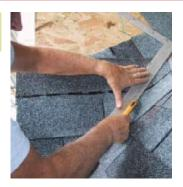
Install the shingles on the dormer side, then use the hook knife to cut the excess shingles. Do not cut into the next layer of shingles. Do this on both sides.
