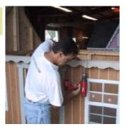
Fasten the 1x3 to the center section using black screws. This will straighten the 2x6 and make it stronger.
