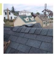
Cut pieces for the ridge cap. See instructions on the shingle package. A regular utility knife will work good to cut this, cut the shingles from the back side. Then install on the top using 7/8" roofing nails.
