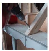
Install the trusses in the premarked spots. Place them to the edge of the 2x6 as the picture shows, not on the gingerbread.
