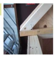
Align, mark by the edge of the 2x3 and put a screw in to hold in place. Note: If there is no mark you can measure in 5.5" and make your own mark.
