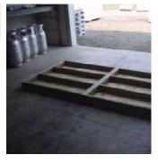
Lay (2) 4x4 flooring sections side by side. Make sure it is on a level area.
