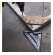
Fasten the truss scabs, keep top even. Install one scab on either side of the truss.
