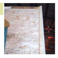
There should be a gap between the 2x2 and OSB like there was on the back side.
