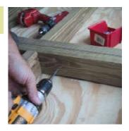
Screw the sections together. Put one screw towards the plywood, and the other toward the top. Put 4 screws on each side roughly 8"-10" apart.
