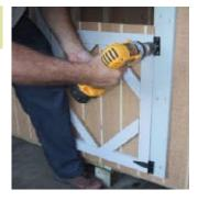
Place the door on the spacer bar. Fasten using only one screw per hinge. This way if adjustments are needed you will not have to undo all of the screws.
