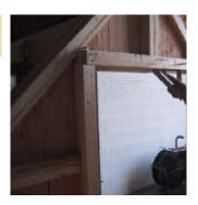
Install (3) 2x3x36" pieces over top of the door and sides over joints. This will provide strength for the door. Keep even with the edge of the door.
