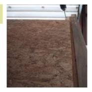
Then fasten onto the edgewall truss. Note the gap between the 2x2 and OSB. The picture shows as it should look. Then fasten onto the rest of the truss.
