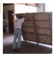
Turn the floor on the back with the plywood facing up. Make certain the ground is level where the floor sets or you may have problems with the panels or roof.
