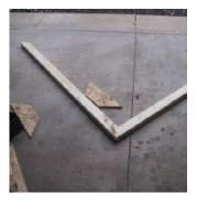
Put the truss angles together. Note: 8x6 angles are the same, but you will need to match the correct 8x8 angles that match the truss scabs. Do not use the rear truss it is slightly shorter.
