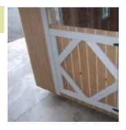
Measure 34" between the door. You may have to loosen back wall slightly to obtain this measurement. Install the top of the door, centering between the top door trim and the bottom half of the door.
