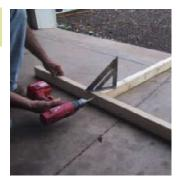
Fasten 2 pieces together to form a T-bar. Use premarked center to make sure it is centered. Make sure to use the correct pieces.
