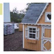
Install the heart window using the small OSB strips. Then install the corner trim using small white nails. Be careful to not "wrinkle" the corners when installing.
