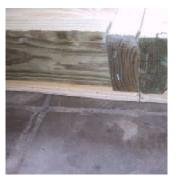
Make sure the plywood is even before fastening! If it is not you will have an uneven floor.
