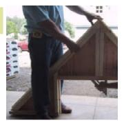
Next fasten panels L&M together. Note keep the edge even. This will be the top of the door so this is very important.
