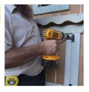
Next install the top door piece. Try to center the door between the header block and the bottom door. If both doors work well, install the rest of the screw and remove the spacer bar. 90
