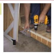
Install the siding beneath the door and put the spacer bar on top. You may have to screw it in place to keep it from sliding away since it is a larger door.
