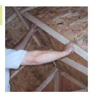
Have someone hold these in place from the inside. Make sure all 3 pieces of OSB are included with the correct angle of the V-brace to the top of the roof.
