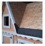
Next cut the tabs off of the shingles and install a strter strip. Use 3/4" roofing nails.
