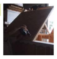
Put 4x4 piece of OSB on trusses. Fasten only on the bottom outside corners. Use black headed screws.
