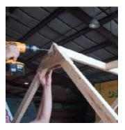
Center the T-bar on the trusses and fasten.
