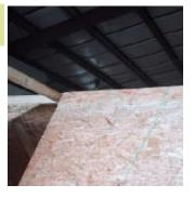
Install the front piece of OSB with angle cut. Note: see how it "shoot's up" into the corner of the T-bar. Next install the top piece.
