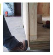
Push the wall in as shown so the siding is against the floor. Fasten the panel to the floor.
