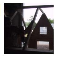
Install the rear truss centered between the trusses and on the T-bar.
