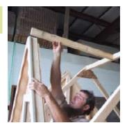
Slide the T-bar piece on top of the dormer, and in between trusses.
