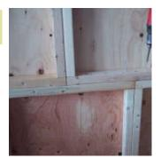
While the other person pushes from the outside, fasten on the inside. Put screws on either side of the splice. Do this on both splices.
