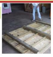
This shows optional 4x4 runners, you will need three in order to have one under the joint. If you use only 2 the floor will sag. Note: these aid in moving the building later, but are optional, unless you are adding the deck & rail, then you MUST add them or the child door will not clear the deck.
