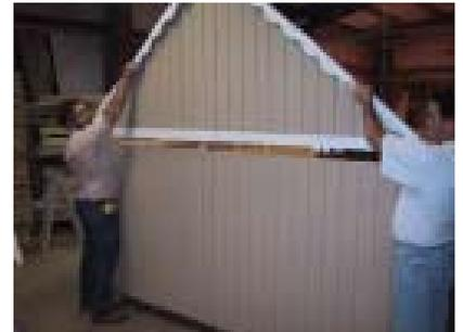
Install these on top of the panels G and H.
