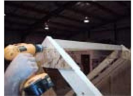
Center the T-bar on the trusses and fasten.
