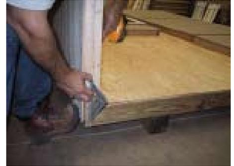
Make sure it is even with the edge of the floor. Push the wall in as shown so that the siding is against the 2x4's on the floor. Fasten the panel onto the floor.
