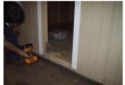
Install small pieces of siding beneath the door. Keep it even with the floor.
