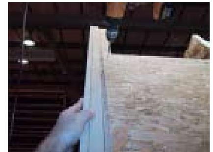
Next install the 4x2 sheet on the front. Note: the same gap between the wall and the sheet as on the back roof.
