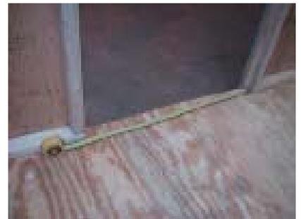
When installing panel L measure the distance between 2x3's. Make sure this measurement is 34". If it is NOT 34", adjust the panels until it is. Otherwise, there will be problems when installing the adult door.
