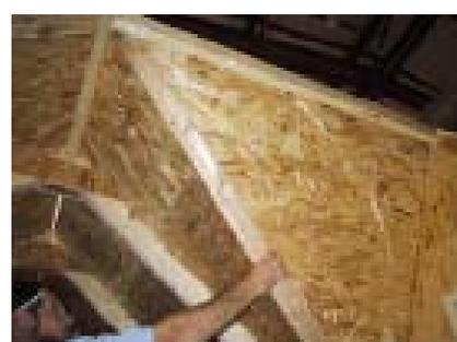
Now have someone hold these in place from the inside. Make sure all 3 pieces of OSB are included with the correct angle of the V-brace to the top of the roof.
