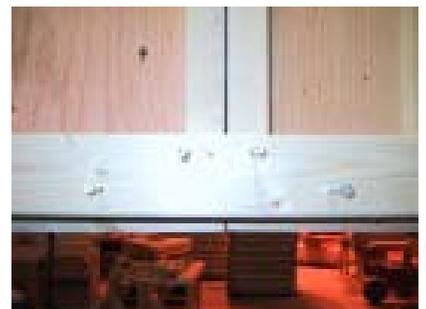
Install 4 screws as shown over the joints.
