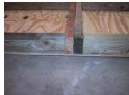
Make sure that the plywood is even before fastening! If it is not you will have an uneven floor, and it could cause problems later.
