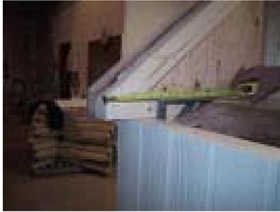
This should measure 5.5 inches from the edge to the inside of the 2x3. The main thing is that it is centered as noted in the previous step.
