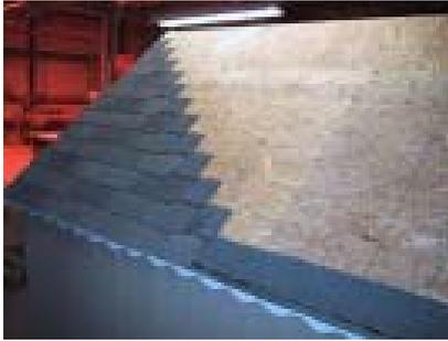
Start installing the shingles as shown and continue until all of the back side is done.
