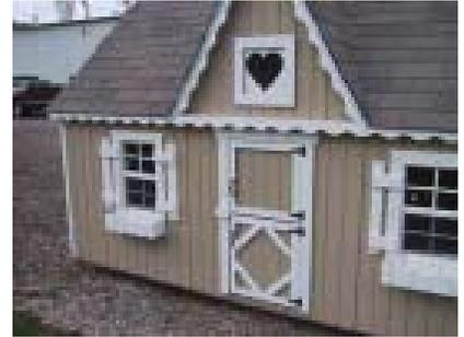
Install the heart window using the small OSB strips. Then install the corner trim using the small white nails. Be careful to not “wrinkle” the corners when installing. Tip: do one side while pressing in, then do the other side.
