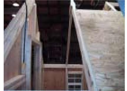
Center the sheet on the other truss that the sheet reaches too. Now fasten this entire sheet, screw roughly 8" apart.
