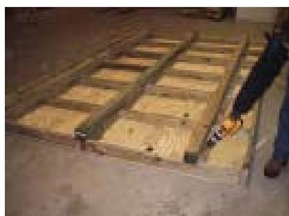
This picture shows the optional 4x4 runners, you will need 3 in order to have one under the center joint. If you use two the floor will sag. Note: these are optional, but will aid in moving the building later. ie: you can put a chain over them and use them to slide over the ground or onto a trailer to move to a different location. If you are adding a deck and rail these are not optional. These allow the small door clearance to open and close.
