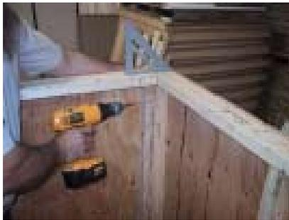
Install panel G. Keep the top even with the other panel. Also remember to keep the siding in against the floor as shown on the first page.
