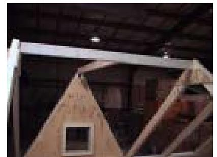
Slide the T-bar piece in the top of the dormer, and in between the trusses.
