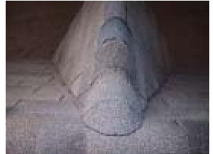
Cut a ridge with a rounded edge as pictured and install.
