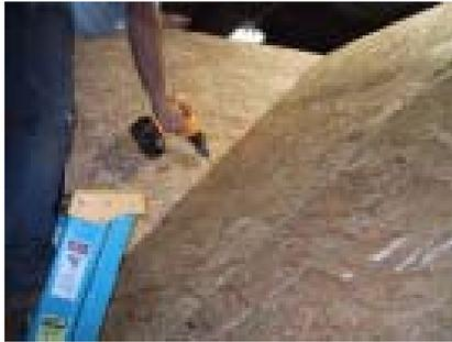
Then fasten using black-headed screws from the top with the other person holding the V-brace.
