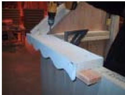
Install the shorter 2x6 with gingerbread, match sets of 4 (8x12) or 3 (8x10) with the numbers and X and O on the pieces.
