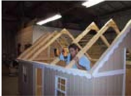
Install trusses in premarked spots. You may have to pull them to the correct position. This is from not fastening the scabs correctly, or from bowing wall or other factors.
