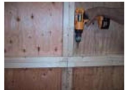
While another person pushes from the outside, fasten on the inside. Be sure to align the top so that it is centered on the bottom wall. Note: the line running from top to bottom. Fasten on all sides of the splice.
