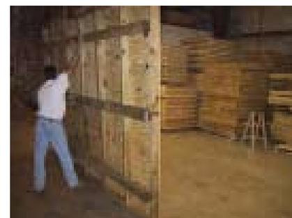
Turn the floor around so that the plywood faces up. Make certain that the ground is level where the floor sets or you will have problems with the panels or the roof. You will need 3-5 people to do this, do this with caution. Do not allow anyone under the section as is shown in the picture.
