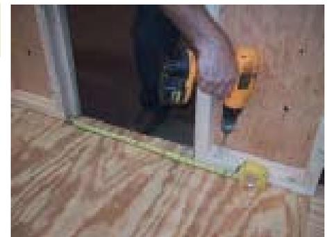
Measure the small door entrance from the 2x3 to 2x3, not the door stop. This should measure 20". Then fasten at the bottom.
