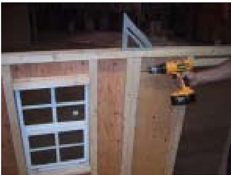
Install panel B. Make sure the top is even with panel A.
