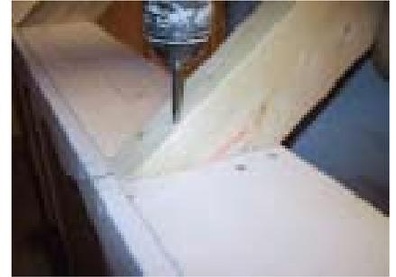
Note: where to place the edge of trusses. Place on the edge of 2x6 and not on the gingerbread.
