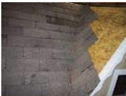
Once you have installed the shingles up the one side, snap a chalk line down the center of the valley.
