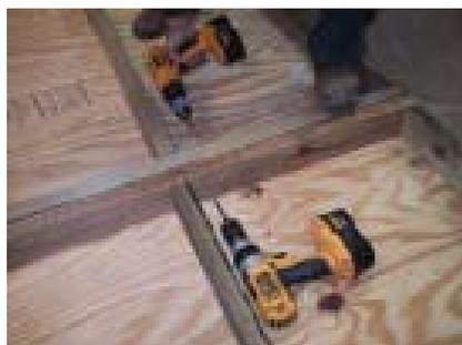
Screw the sections together. Put two screws in from each side for a total of 4 screws, one towards the plywood and one towards the top. Repeat this roughly 8-10 inches apart.
