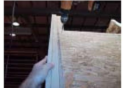
This shows what the edge of this sheet will look like on the end wall. Note: the gap between the wall and the sheet.
