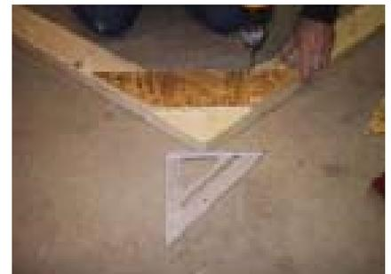
Fasten the truss scabs, keep the top even. Install one scab on either side of the truss. Make sure the scab does not stick out past the truss.
