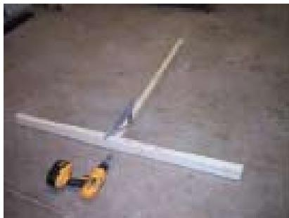
Next fasten two pieces together to form a T-bar. Use the premarked center to make sure it is centered. Make sure to use the correct pieces. These are 2x3's.
