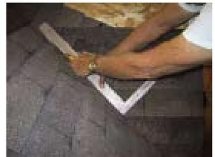
Then install the shingles on the dormer side, then use a hook knife to cut the excess shingles. Do not cut into the next layer of shingles or the roof may leak. Repeat these steps on the other side.
