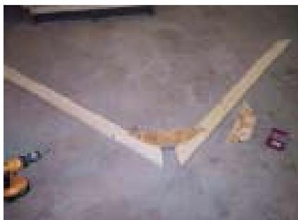
Put the truss angles together. Note: you will have to match the correct angles that match the truss scabs. Do not use the rear truss (if shorter).
