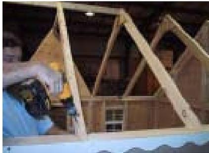
Center the rear truss between the trusses and on the center of the T-bar.
