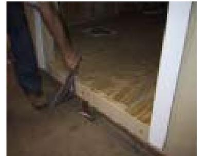
Install the siding beneath the door and put the spacer on top. You may have to screw it in place to keep it from sliding since it is a larger door.
