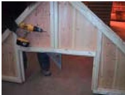
Next fasten panels M & N together. Note: Be sure to keep the edge even. This will be the top of the door so this is very important. The trim should go to the bottom as can be seen in the picture below.
