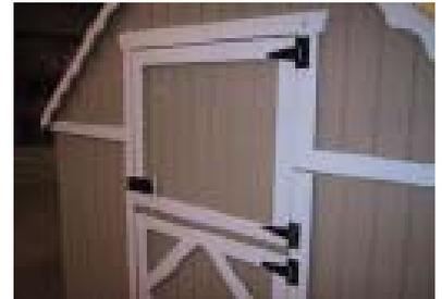
Install the top of the door, centering it between the top door trim and the bottom half of the door. Install the latch.
