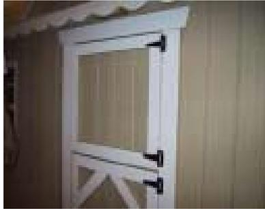
Next install the top dormer piece. Try to center the door between the top trim piece and the bottom door. If both doors work well, install the rest of the screws and remove the spacer bar.
