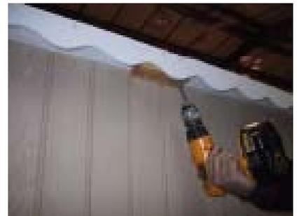
Once the last piece is in place, fasten the blocks underneath to the other piece. This will make the wall and 2x6s sturdy. Repeat the steps on the other side.
