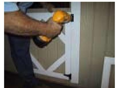
Place door on the spacer bar. Fasten using only one screw per hinge. This way if you need to make adjustments you will not have to undo all the screws.
