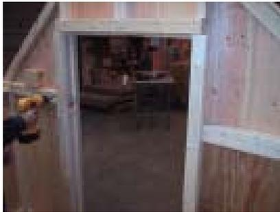
Install (3) 2x3x36 pieces over the top of the door and sides over the joints. This will provide strength for the door. Keep even with the edge of the door.
