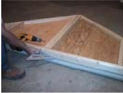
Fasten panels I and J to each other. Make sure they are even on the bottom. Piece may bow slightly; this can be made straight in the following steps.
