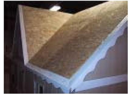
Next install the drip edge (this should have been purchased by the customer at a local home improvement store). You can use tin snips or sidecuts to cut the drip edge and make cuts so that it fits on the angles of the roof. Fasten with 3/4" roofing nails.
