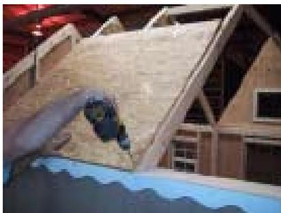
Put a 4x4 (8x12) or a 3x4 (8x10) piece of OSB on the trusses starting with the rear truss. Use black headed screws. It is VERY important to put the roof together correctly, also if your foundation was not level it will show up here!
