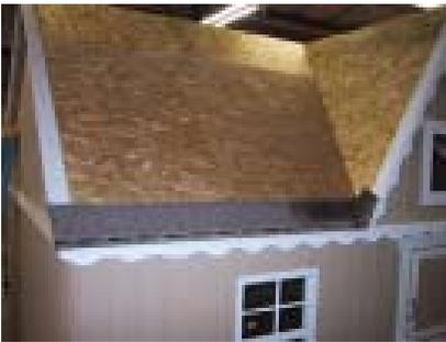
Cut the tabs off of the shingles and install a starter strip. Notice the glue strips toward the bottom. Fasten with 3/4" roofing nails.
