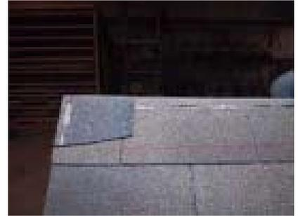
Cut pieces for the ridge cap. See instructions on the shingle package. A regular utility knife works well for this, cut the shingles from the back side. To start with, cut one into a smaller piece as shown. Then install on the top using 7/8" roofing nails.
