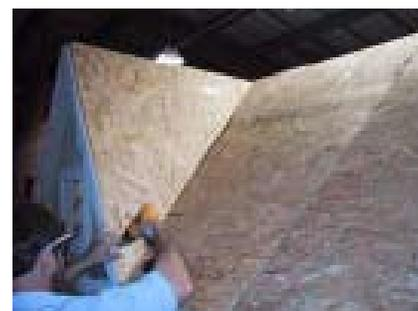
Install the dormer pieces. Refer to the sheet to see the size. Now install the dormer piece and fasten. Then repeat the steps on the other side of the dormer.
