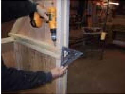
Keep the edge of the door frame even and push the trim in against the siding and fasten.
