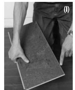
This space must also be provided at all columns, heating pipes, steel doorframes, etc. The planks are laid with the tongue side facing the wall to be able to work with the tongue/groove system.
