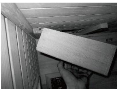
FIG 15.2 Installing the Radio Wood Housing
