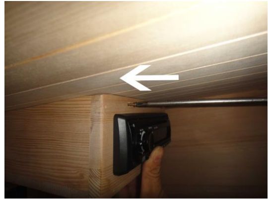
FIG 15.4 Screw wood housing to sauna room
