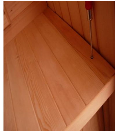
FIG 10 Securing Benches with screws
