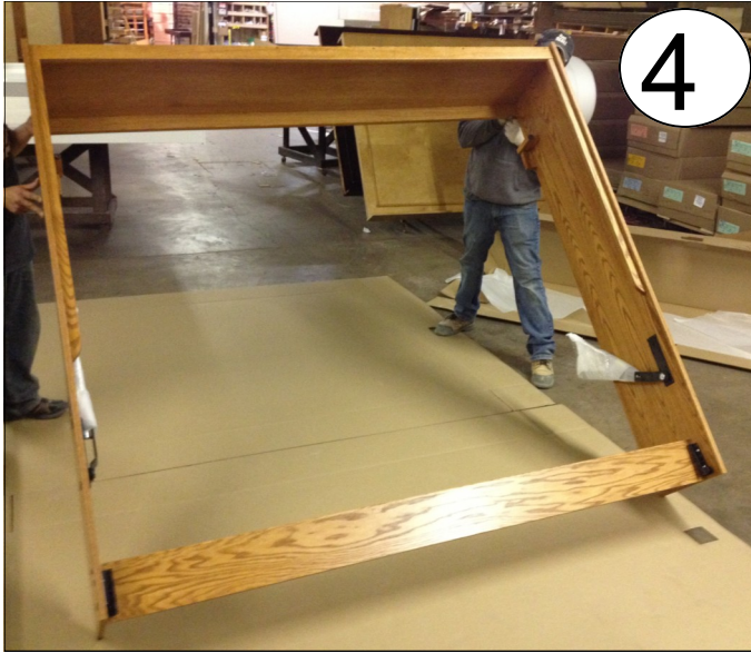
Stand assembled cabinet up in front of , but out away from the wall.
