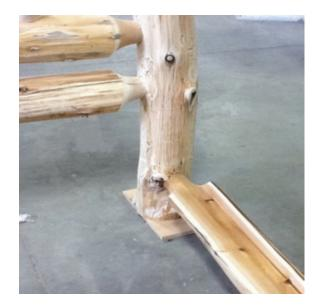
5. When rails are correctly installed, the short flat-edge should be aligned vertically as seen below.
