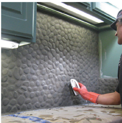
Sweep out more grout with a brush
